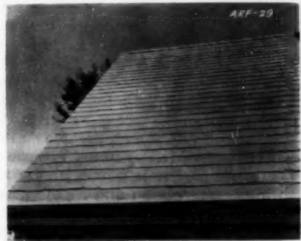
Molded asbestos shingles, used by the millions for fireproofing and beautifying modern homes. (Courtesy Johns-Manville).
